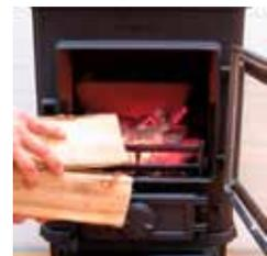
The stove door should normally be opened gently the first 2 - 3 centimetres, then you should wait until the pressure has equalised before opening the door all the way. This technique will prevent smoke from getting out, particularly when there is a poor draught. The stove door should never be opened when the stove is being fired vigorously.
