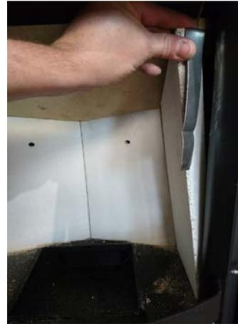
*Carefully lift out both side fire bricks, ensuring the securing clip remains with the brick.
